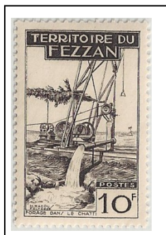
2N18 Drilling for water
