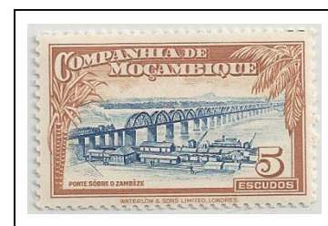
191 NH Zambezi Railroad Bridge
